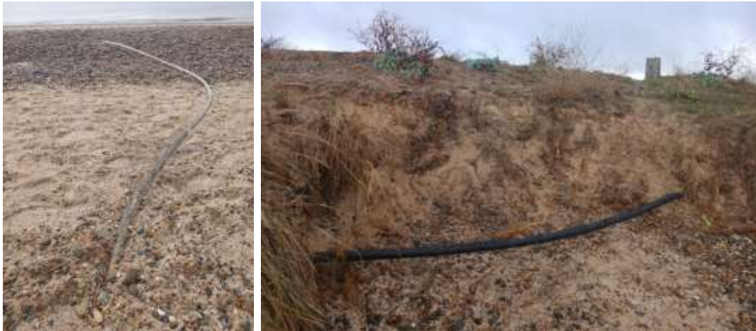
Figure 1: Photos of cables exposed at Pakefield from Storm Amy inspection by ESC Coastal Management Team (14-10-2025).
